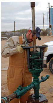
Install stuffing box protector
